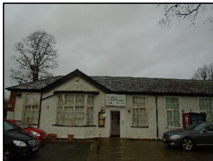
Plate 1: showing a typical view of the Club House. Photograph looking at south eastern elevation.
