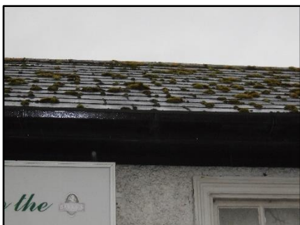
Plate 3: showing a typical view of the Club House roof cover.
