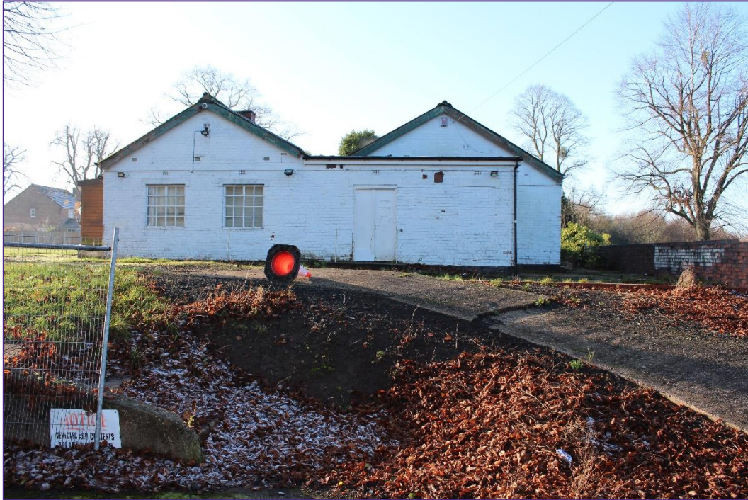
Plate 15: East gable ends of changing room extension viewed from car park.
