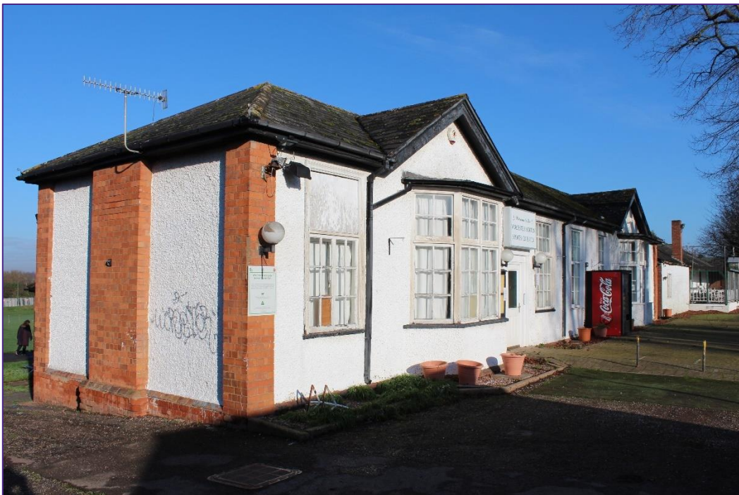
Plate 8: View east over Clubhouse with evidence of chimney breast noted on end flank.
