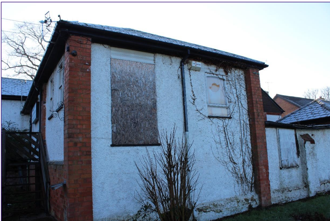
Plate 12: Boarded up windows on north flank of Clubhouse rear wing and later fire escape and staircase (left).
