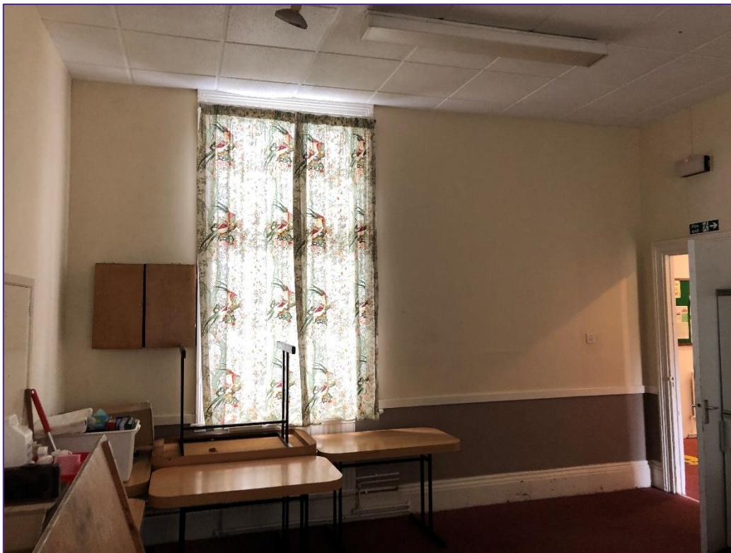
Plate 22: Remaining part of subdivided left-hand room on principal range (Photo courtesy of Greenwood Projects).
