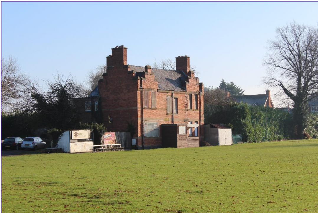
Plate 26: The Stewards' Houses viewed from edge of Site with later extensions noted to rear.
