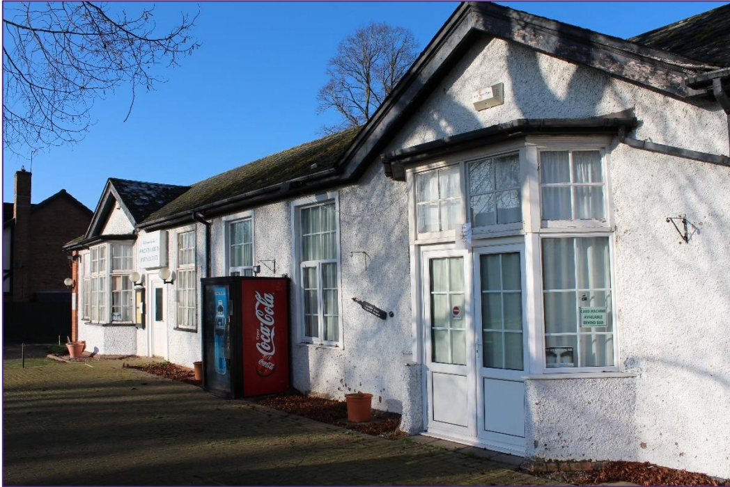
Plate 7: Front elevation of Clubhouse with evidence of later PVC windows.
