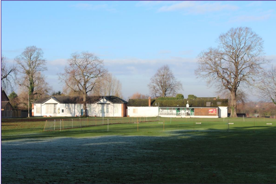
Plate 1: The Clubhouse with later changing rooms (the 'Site') added to right hand side viewed south from sportsground
