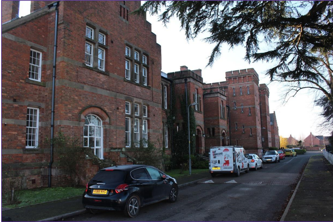
Plate 23: The former Keep (right) and flanking wings viewed from edge of sports ground.
